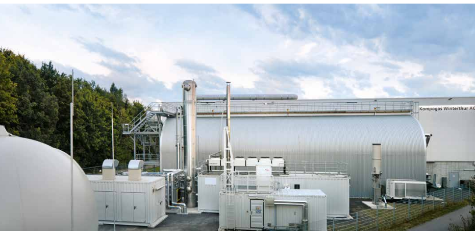
Kompogas® plant with HZI BioMethan treatment technology in Winterthur, Switzerland
